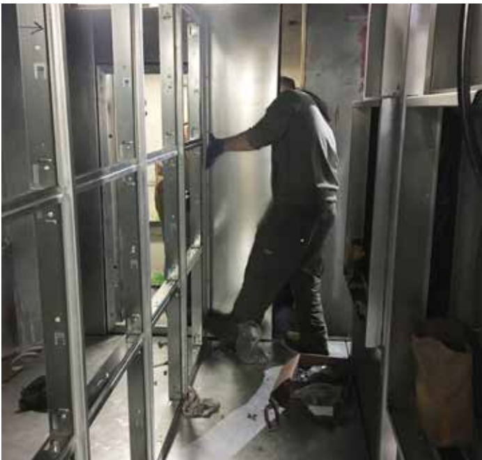
Assembling the panels on the framework of the ACCESS air handling unit
